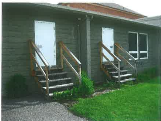
Egress doors at 1966 building
