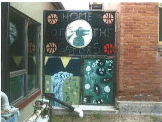
Fire Escape – Security Gate Looking West
