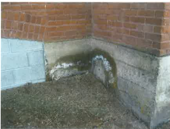
Foundation- Northeast corner of porch.
