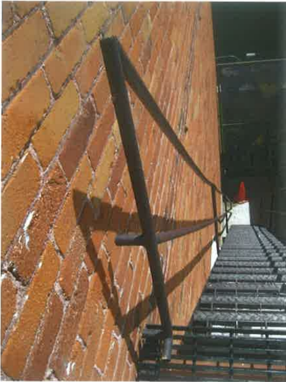
Fire Escape – Looking East
