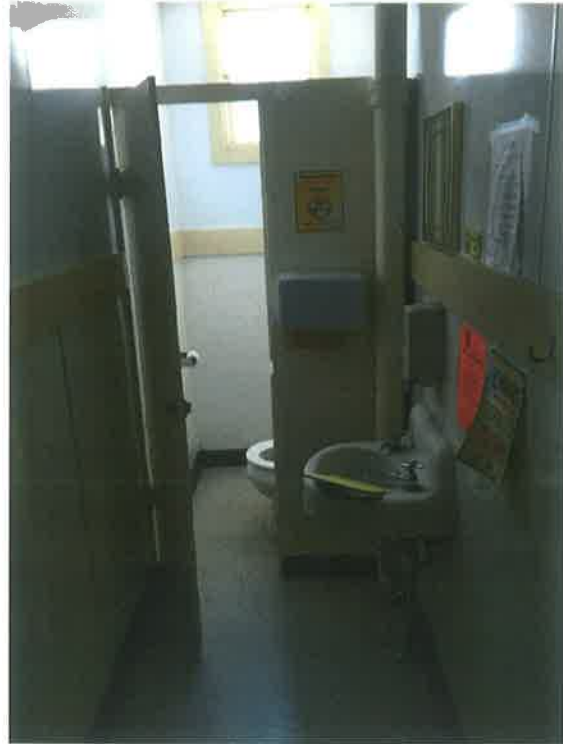
Toilet Rooms – 1 st Floor Women's Room
