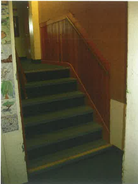
Stair - Mid-landing to First Floor
