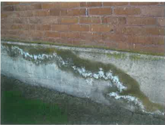
Foundation - North wall east end.
