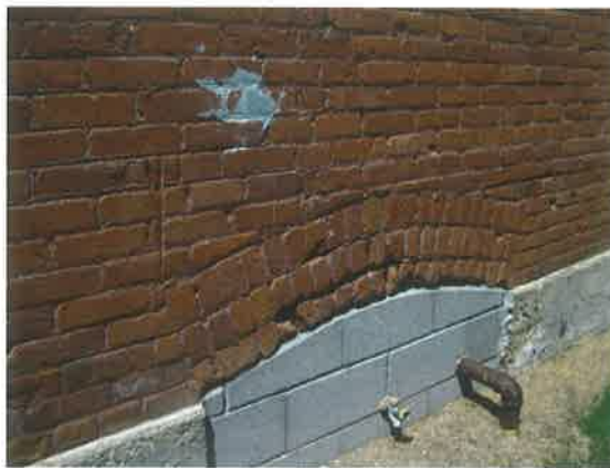
Masonry Wall - East elevation.
