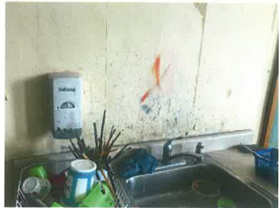
Interior Walls - Art Room west wall.
