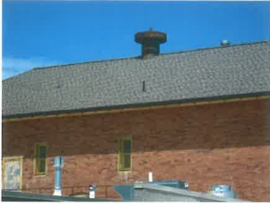
Roof - South facing slope.
