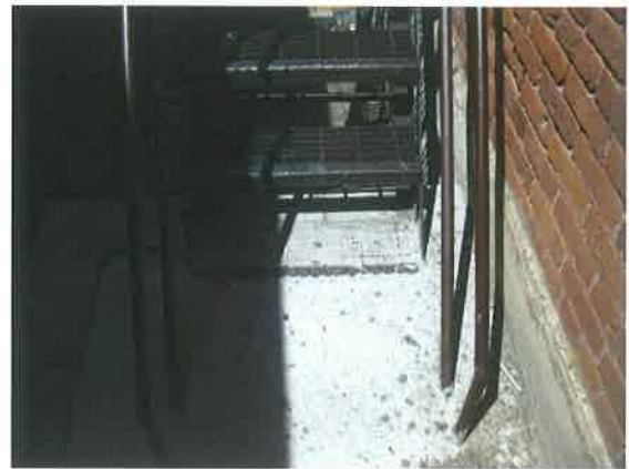
Fire Escape - Landing
