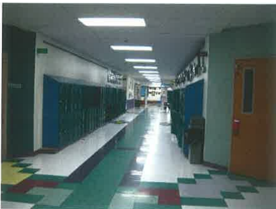
2003 addition corridor looking east
